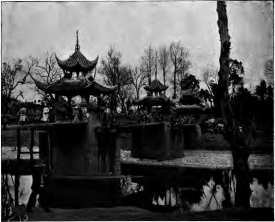
Bridge on the Chengtu-Tibetan Road, crossing irrigation channel— partly natural, partly artificial.
